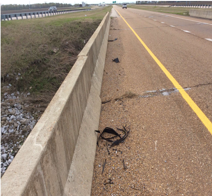
PHOTO 1 Description Gutters are full of dirt and debris with vegetation growing.
