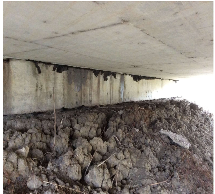
PHOTO 2 Description Abutment 1 cap undermined
