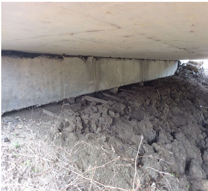
PHOTO 3 Description Abutment 2 cap undermined.
