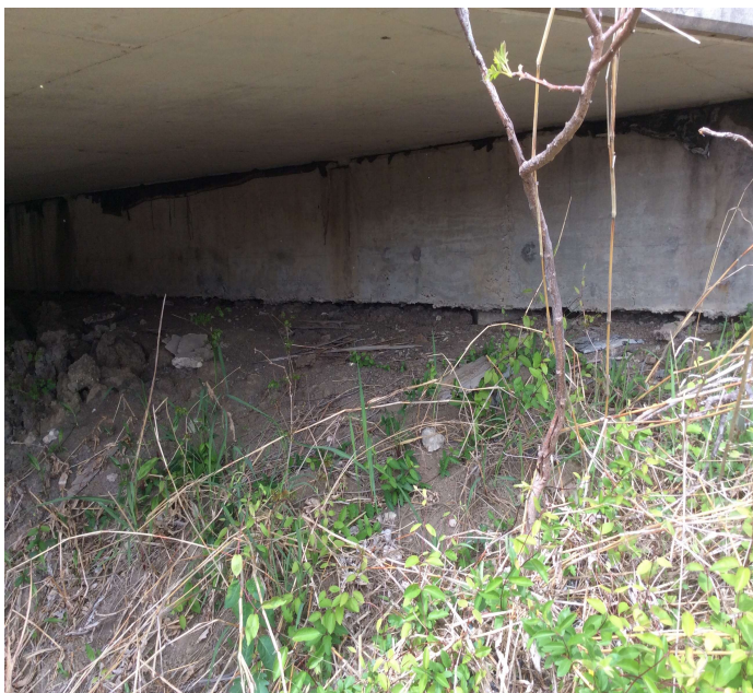
PHOTO 4 Description Abutment 1 cap undermined.
