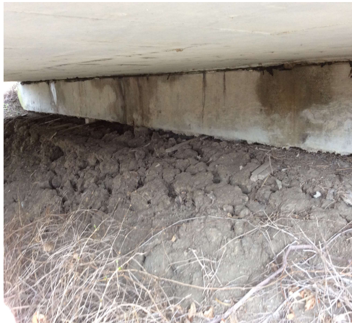
PHOTO 1 Description Abutment 2 cap undermined
